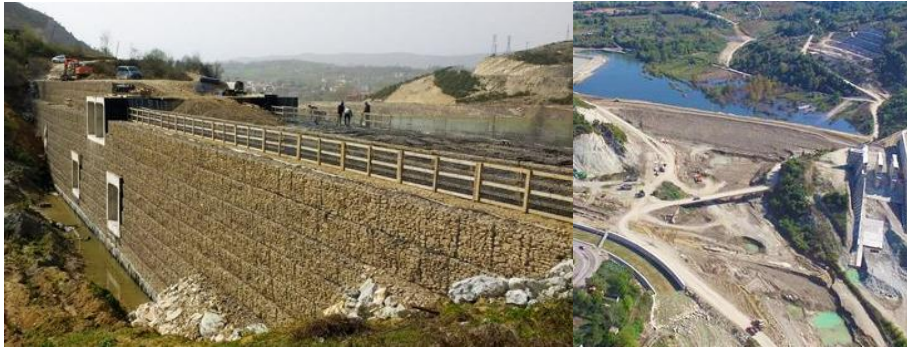
Embankment Manufacturing of Kozcağız Dam-Gabion Basket with Terramesh System [14]
