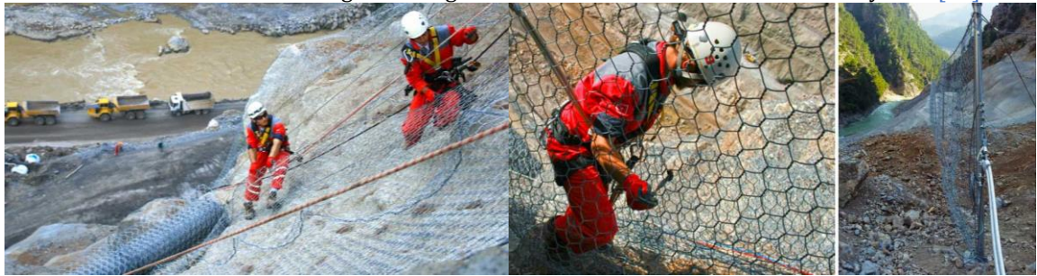
Rock Barrier and Steel Grid Application of Kavşakbendi Project- Gabion Wire Mesh [15]
