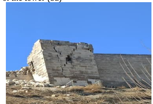
with possible torsional effects if the tower is asymmetrically connected to the walls, shear cracks in the upper part of the tower (3b)
