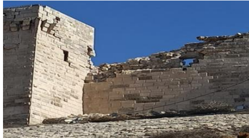
Figure 3. Types of damage (2a), (2b) and (2c) on the walls of the castle
