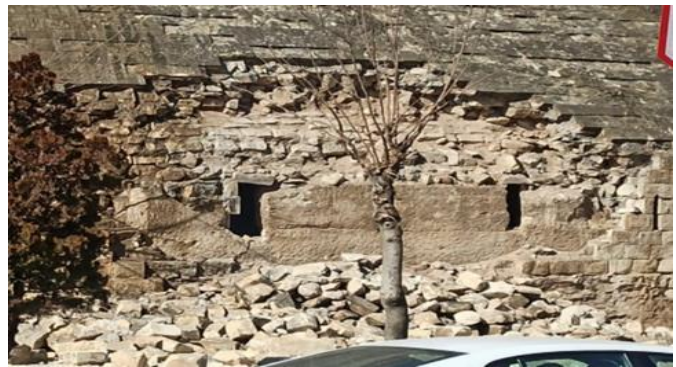
delamination of the cladding (1b)
