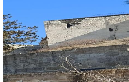
cracks caused by the different dynamic behavior between tower and wall (2a),
