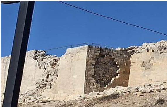
crumbling of masonry (1a)
