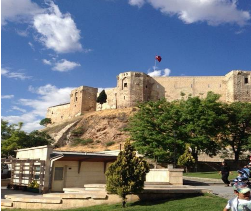
Figure 1. Gaziantep Castle before the 2023 Gaziantep-Kahramanmaraş earthquakes
