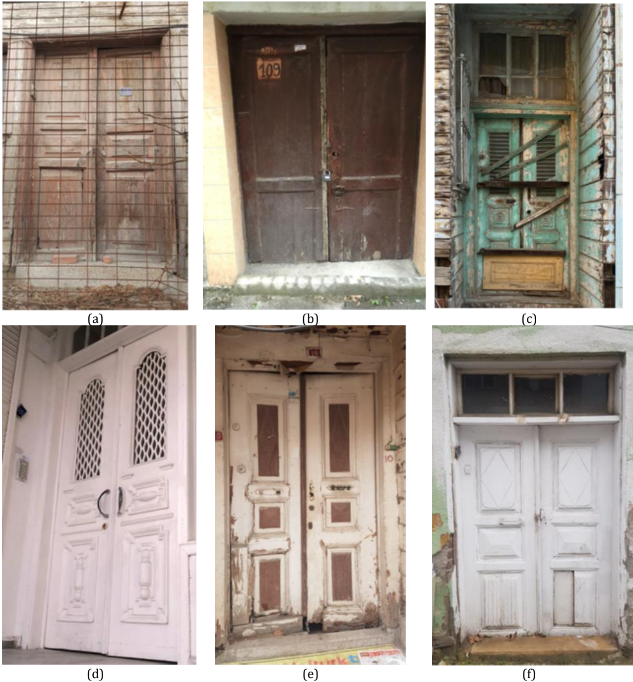
Figure 3. (a) Example of the plain door with a panel, Muratlı Road number: 27, (b) Example of the plain door with a slat, Peştemalci Road number. 109 (c) Example of an ornate door with a skylight, Tintinpinar Road Number: 7, (d) Example of an ornate leaf door, Rakoczi Road No: 26, (e) Example of an ornate door with different decorations in different colors, Muratlı Road Number: 12, (f) Example of an ornate door with a skylight, Muratlı Road Number: 22
