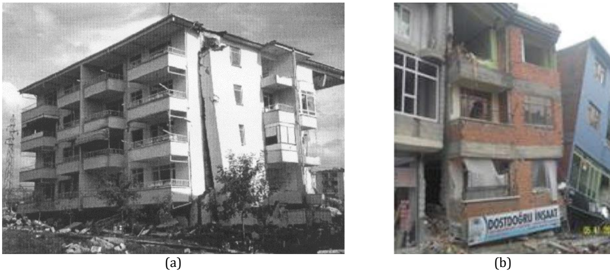
Figure 2. Some examples of soft story damages, (a) a building having its first two stories damaged under 1999 Kocaeli earthquake, Türkiye [5], (b) a building damaged under 2011 Van earthquake, Türkiye [6]
