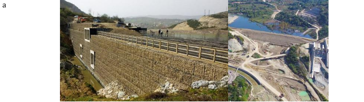
Embankment Manufacturing of Kozcağız Dam-Gabion Basket with Terramesh System [14]
