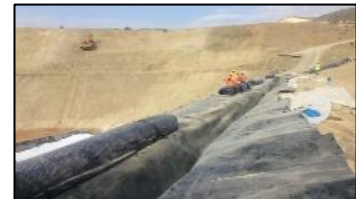
Figure 5. The anchor trenches
