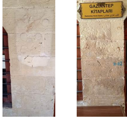
Figure 4. Anthropogenic deteriorations in Historical Gümrük Inn
