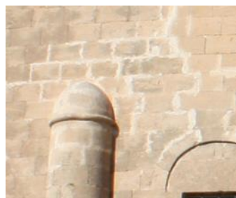
(b) Use of cement
