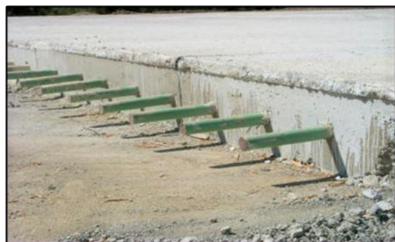
Figure 3. Dowel bars used in transverse joints
