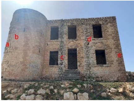
Joint discharge (a), Cement use (b, c), Surface loss (d), Color change (e)
