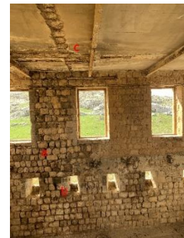
Joint discharge(a), Color Change(b), Piece Loss(c)
