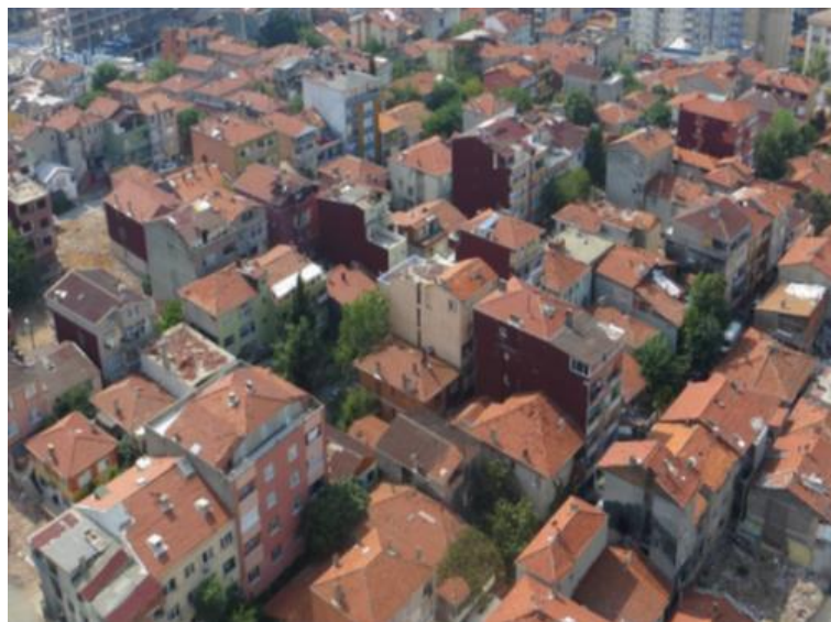
Figure 3. Structuring of Fikirtepe before the Urban Transformation Project [20].
