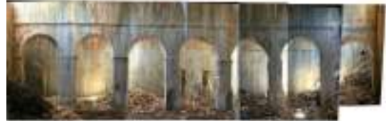
Fig.9-Longitudinal view of the arches in the Cistern
