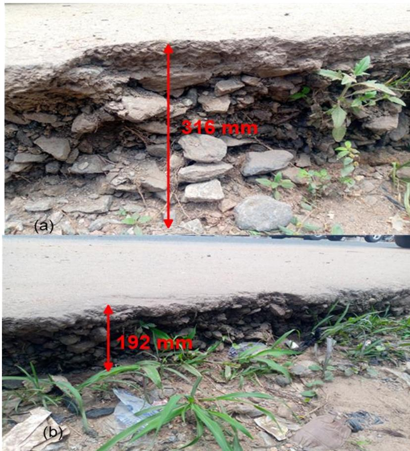
Figure 12. Sections of the Highway Structure Exposed along the highway edge/shoulder from which existing design thickness was measured (a) weak subgrade segment (b) good subgrade segment
