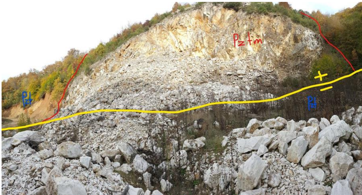
Figure 7. The general view of the NW-SE trending dip-slip fault cutting the Calcite Quarry (Looking from the Southwest to the Northeast). Abbreviations: Pzt; Torasan formation, Pztm; Marble Member
