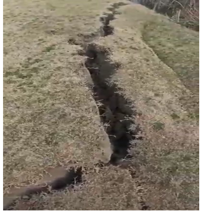
Figure 7. Hemite Village Surface Fault Fracture.
