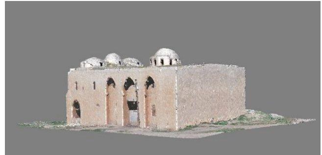
Figure 3. The generated point cloud
