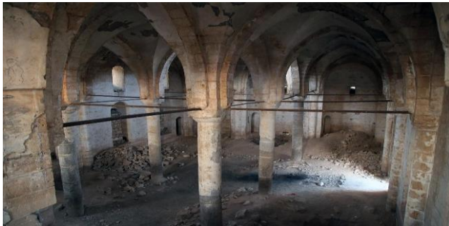
Figure 6. Interior view of Germus Church
