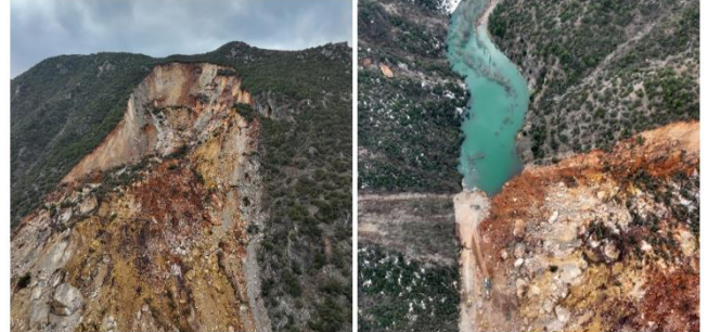
Figure 1. A general view of landslide area
