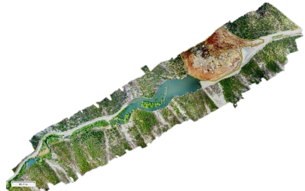
Figure 6. Calculation of the approximate volume and the spread area of the landslide
