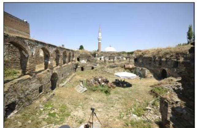
Figure 3. Lutfu Pasa Hami during laser scanning of the inner courtyard
