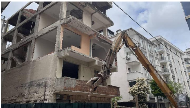
Figure 1: Urban Transformation Application Demolition Study (URL_3)
