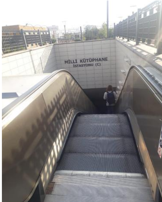
Figure 4. Ankara National Library Underpass
