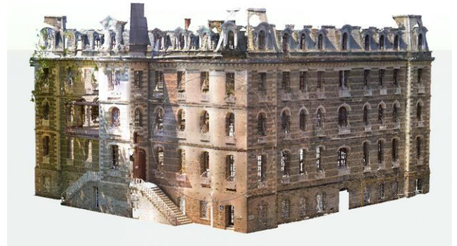
Figure 5. 3D point cloud model of the 1 st Men's Dormitory buildings
