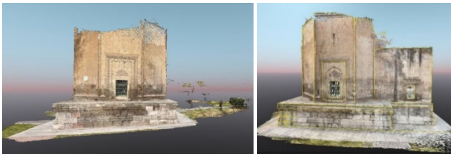
Figure 9. Unpurged and purged Ali Cafer Kumbet point cloud data (East facade).
