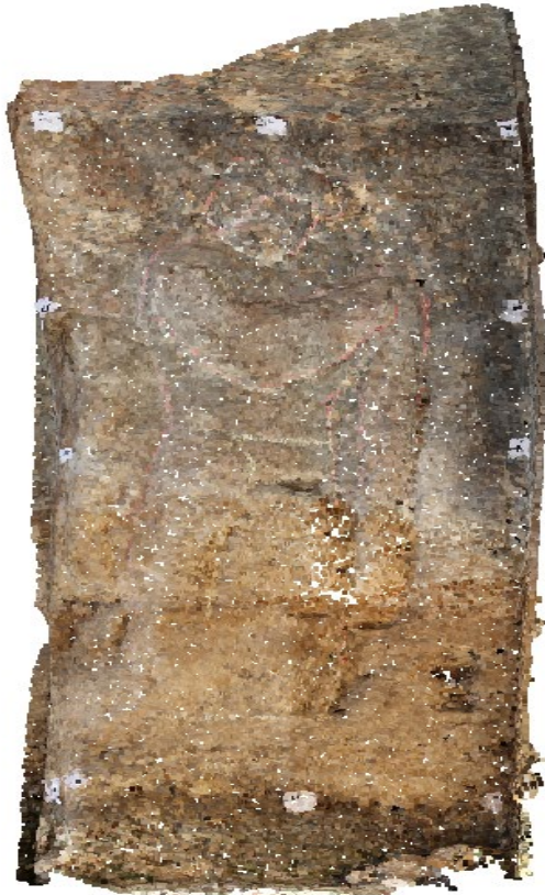
Figure 7. Point cloud obtained by LIDAR scanning.
