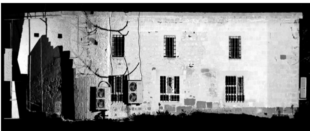
Figure 8. Orthophoto of west frontage
