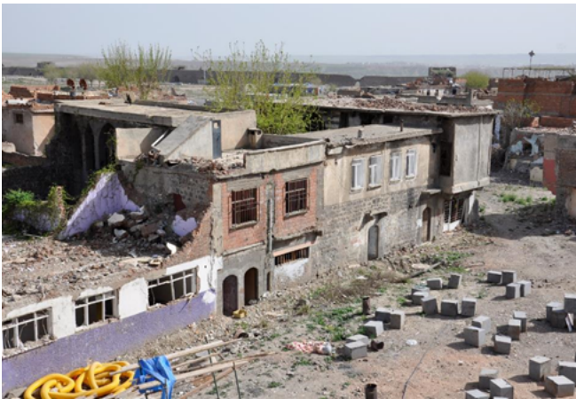
Figure 2. Current state of the building
