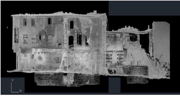
Figure 8. Orthophoto of the south façade
