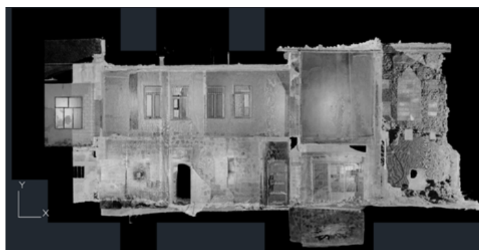
Figure 8. Orthophoto of the western façade
