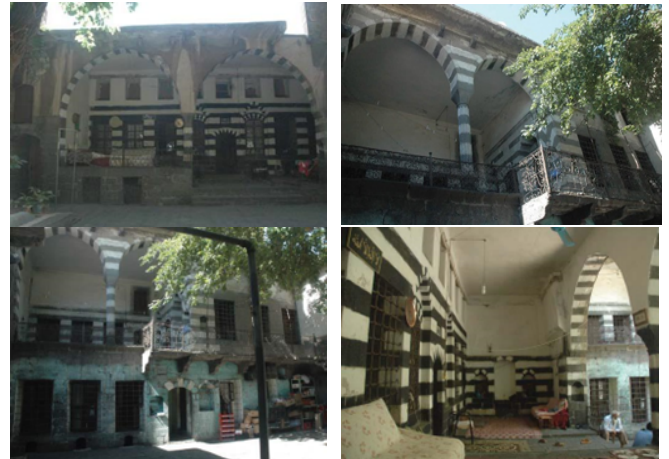
Figure 3. The original state of the building
