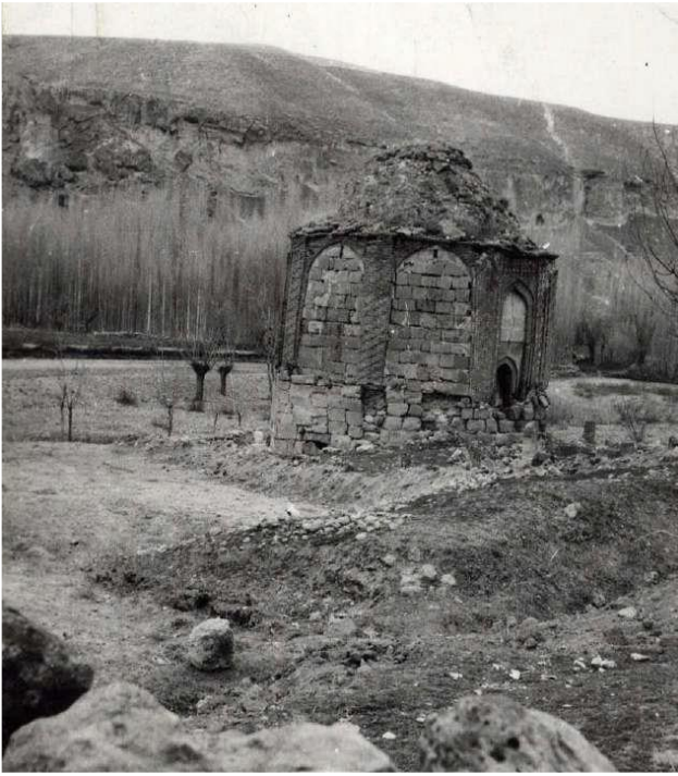
Figure 5. Structural deformations of Tomb around 60's.
