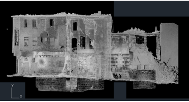
Figure 8. Orthophoto of the south façade
