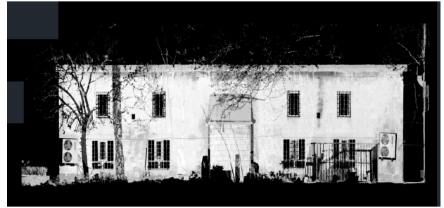
Figure 10. Orthophoto of south frontage
