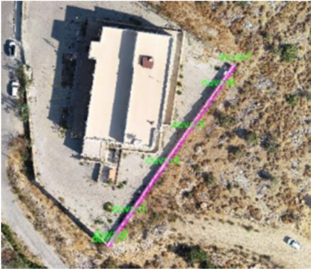
Figure 11. SGK Building and Wall Measurement
