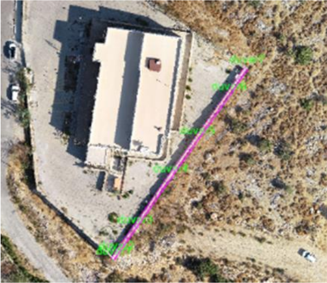
Figure 11. SGK Building and Wall Measurement
