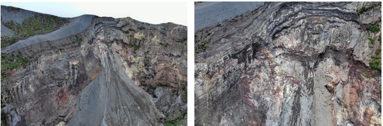
Figure 30 & 31 - Rockfall formation left from the 2019 material release and resulting sieche September 2022
